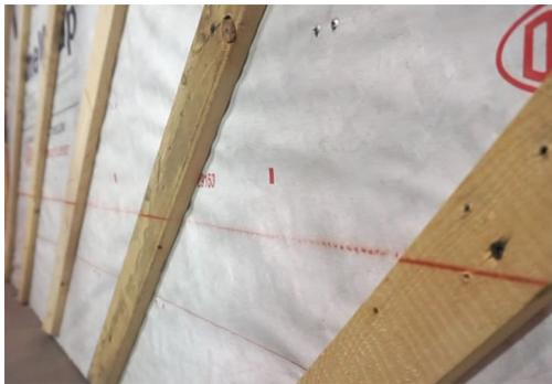
Now, fix the M10D starter strips 3 inches above where you want your wall to begin. Use flathead MAC Anticorrosion Wood Screws or MAC Anticorrosion K-LATCH Screws (1 1/8 or 2 1/2 in). Secure the strip using one screw. When you are level, screw it in place.
