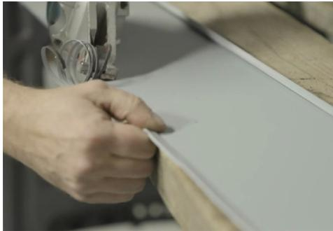
If the plank isn't flush with the height of the wall, place the extra piece backwards onto the J-Trim moulding, M01C to add support to the plank that was cut.
